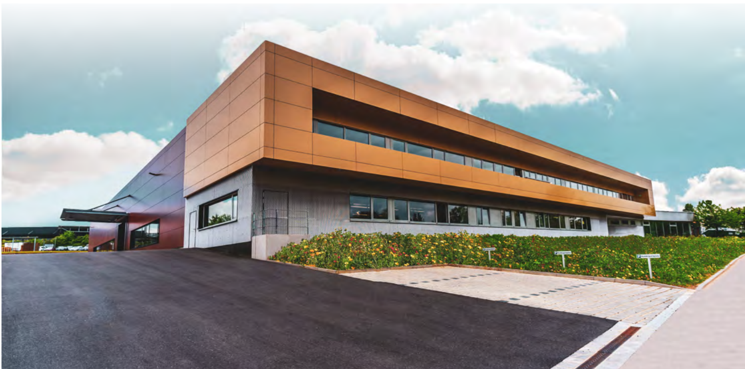
Headquarters of the syskomp Group, Amberg
